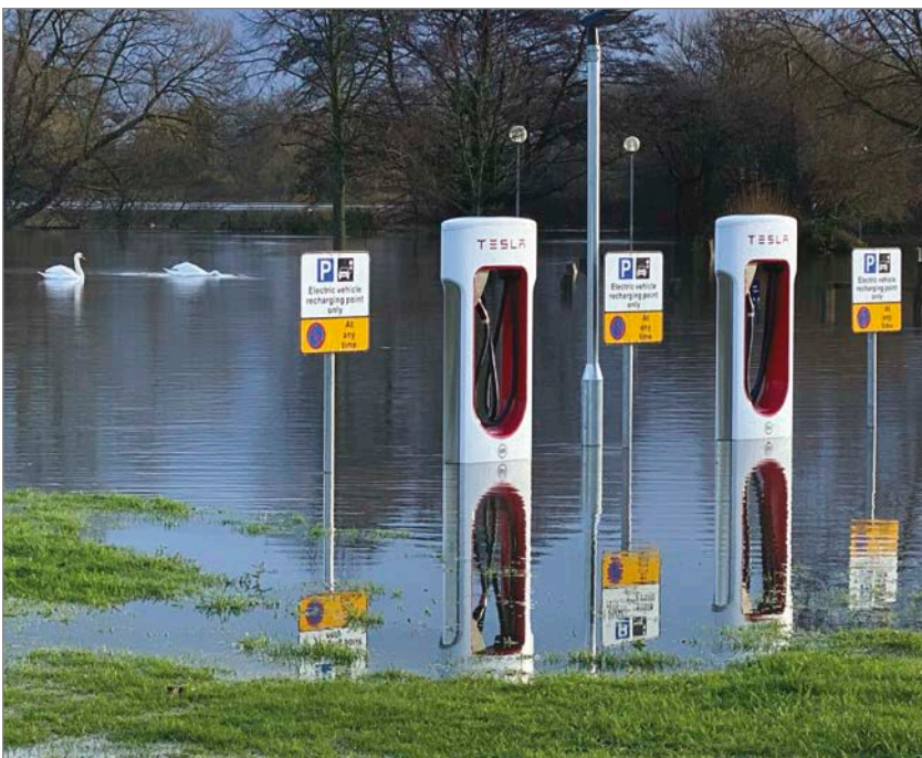
Tesla car charging points at Sindlesham, UK, underwater owing to heavy winter rain (photo: Phil Creighton, Editor of The Wokingham Paper ; see https://is.gd/teslaflood for more).
